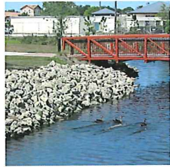
Moore's Creek Existing Site Improvement Photos
