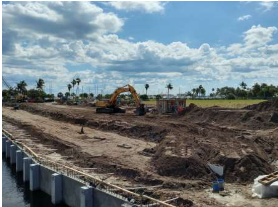
Subject – SE view from Moore's Creek bridge
