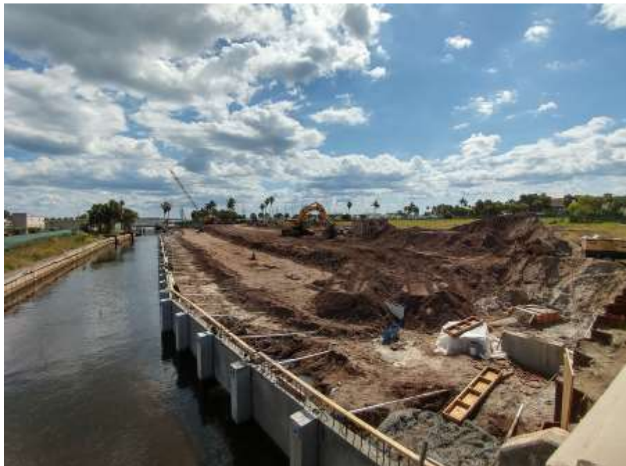
Moore's Creek & bulkhead installation in progress
