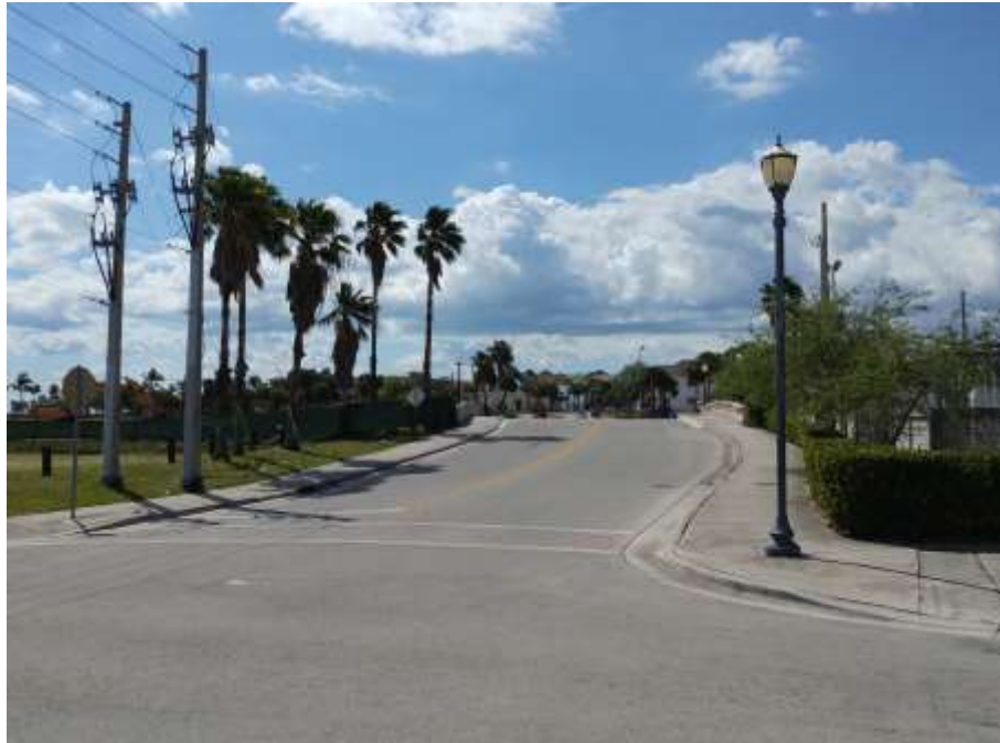
Southerly view along N. 2 nd St. & Moore's Creek bridge
