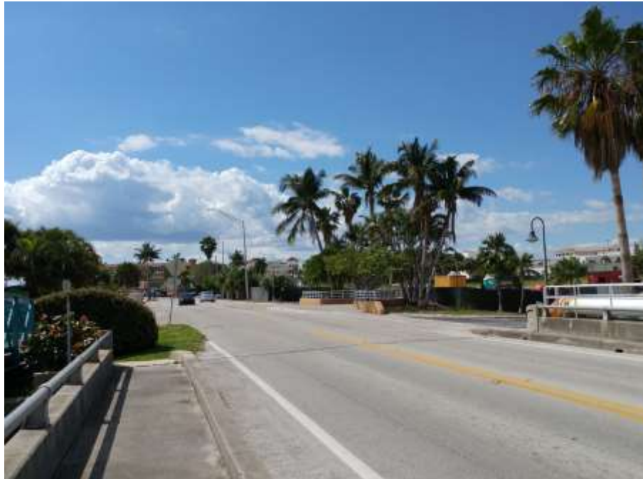
South view subject's Indian River Dr. frontage (right beyond bridge railing)
